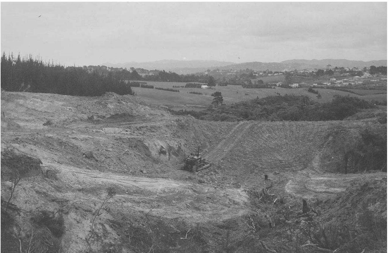
Bulldozer at work in the dam.
