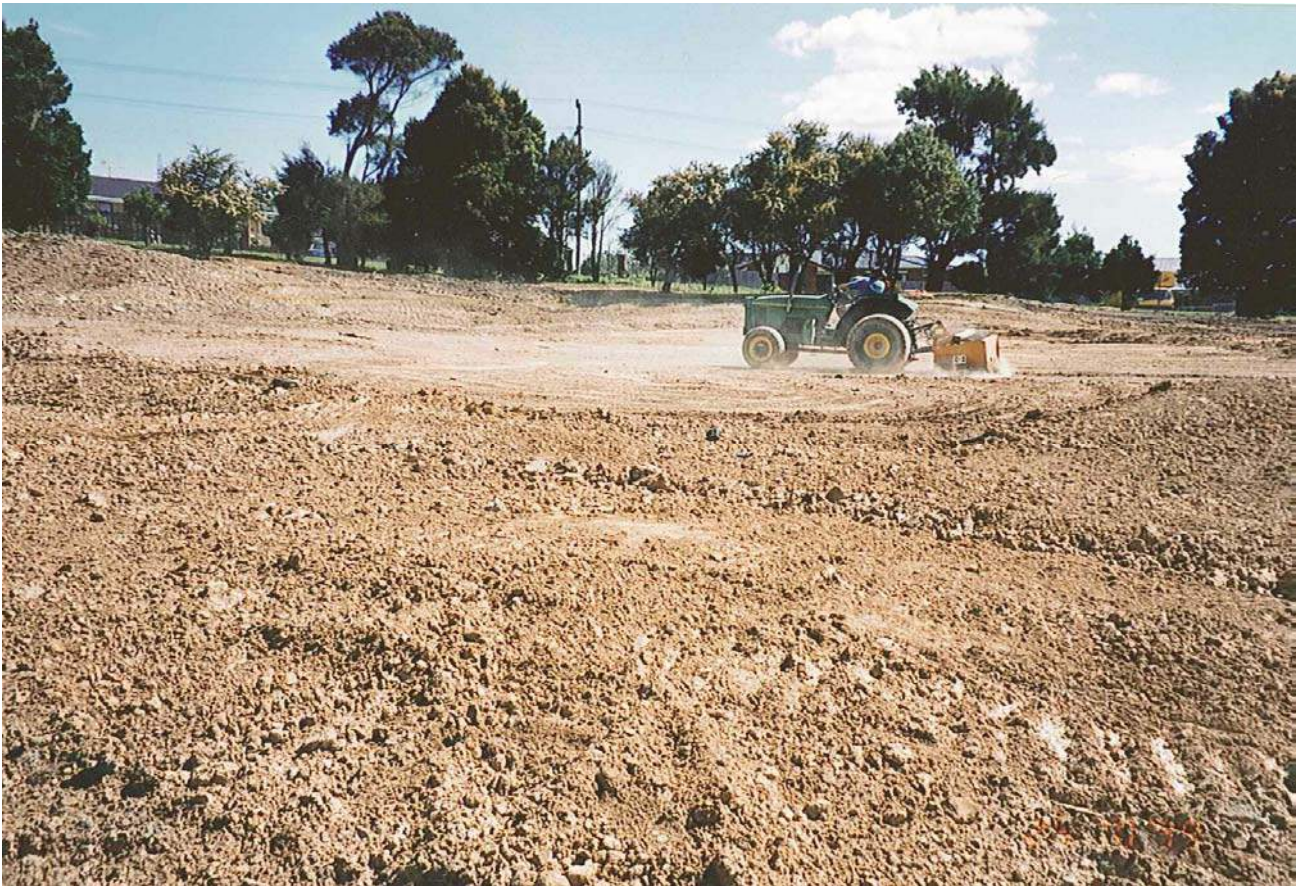
Building the new 13 th green, 1999
