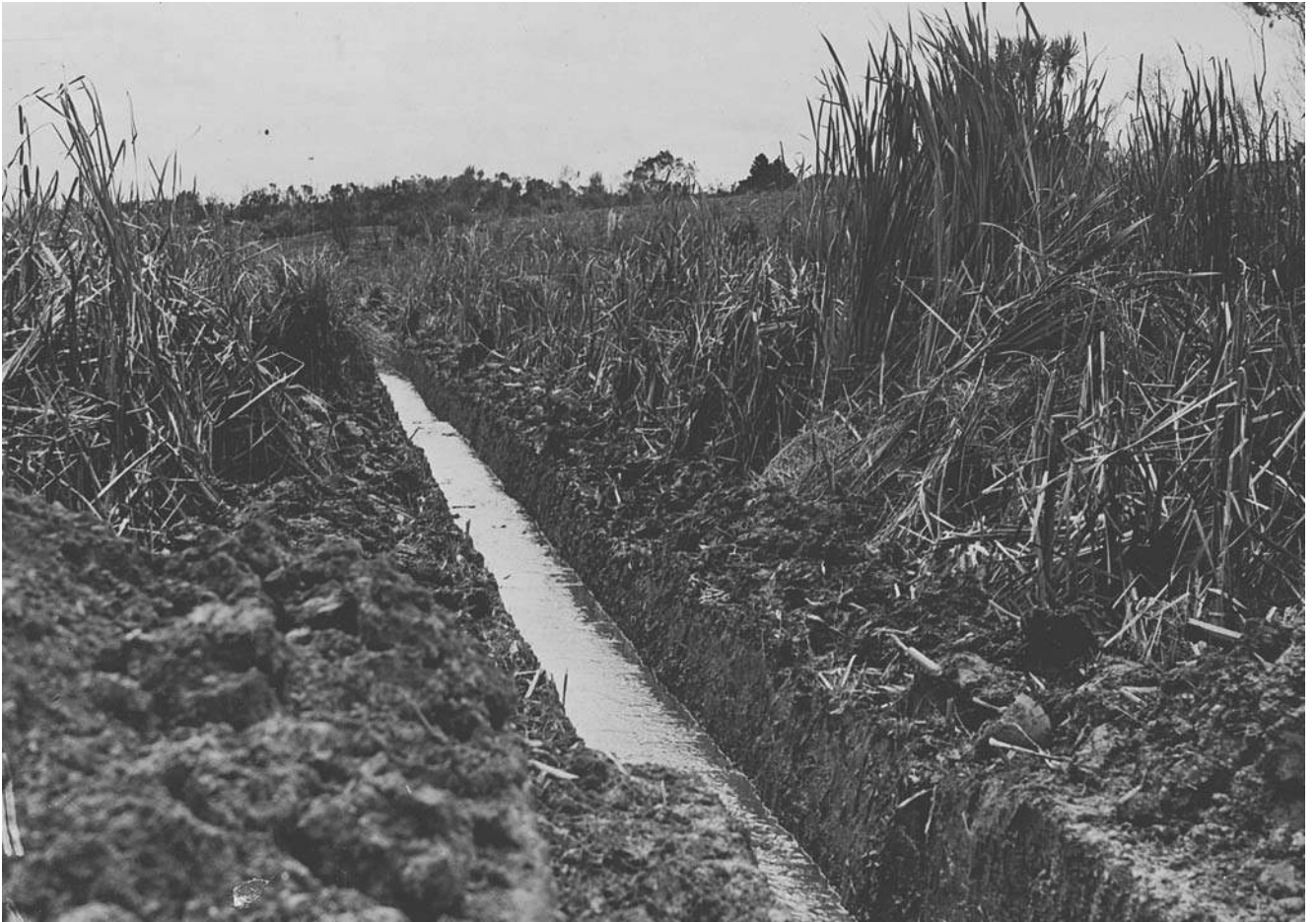
Hand cut drain through Raupo Swamp
